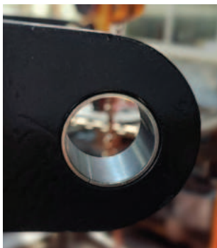
LOW MAINTENANCE BUSHES AND CHROMIUM PLATED PINS.
